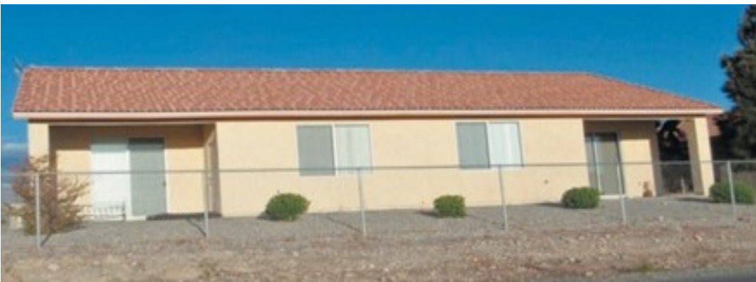
Photo 4. House with its exterior west wall unshaded. Summer cooling costs are much greater than if that wall were shaded with an evergreen small tree.
