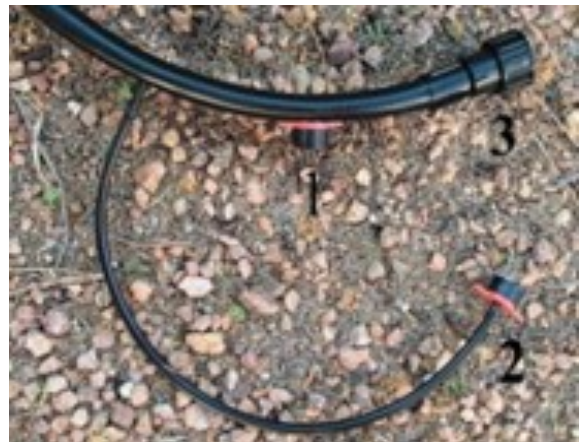
Photos 57 and 58. Drip tubing (left) showing the opening of an embedded drip emitter for the release of a precise amount of water in Lph or gph. Single emitters (right) can be connected to blank tubing, either directly (1) or by attaching them to one-quarter-inch distribution tubing (2). An end cap can be removed to flush the blank tubing which helps prevent plugging (3). (Photos by R. Morris.)
