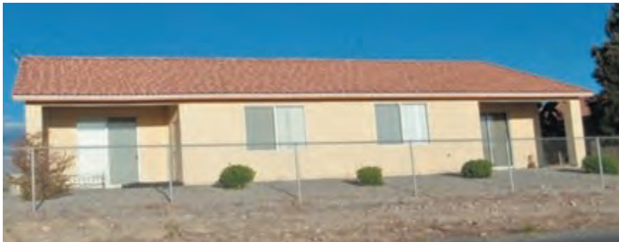
Photo 4. House with its exterior west wall unshaded. Summer cooling costs are much greater than if that wall were shaded with an evergreen small tree.
