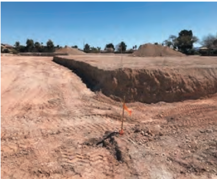
Photo 2. New residential site in Las Vegas, where almost three feet of soil taken from a distant location was used to create a new elevation for both the yard and foundation. The light tan color of the soil indicates low organic content. (Photo by D. Devitt).
