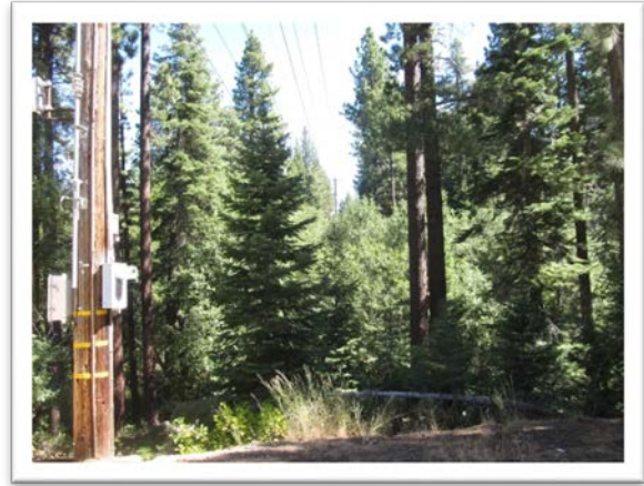
Picture is before treatment along 160 KV power transmission line at Van Sickle Bi-State Park.
