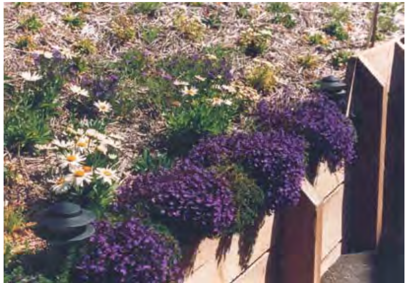
A close-up of the retaining wall on Page 17 (top). The wall mechanically stabilizes the eroding cut slope. The roots of native daisies, columbines, lupines and delphiniums hold soil in place. A layer of organic mulch over the soil improves infiltration.
