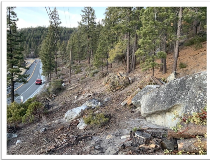
Hand Thinning of the East Shore Project - Zone 1, as part of the Lake Tahoe Powerline Resilience Corridor Project.
