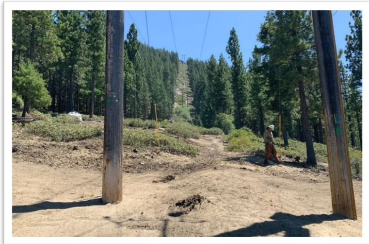
Fuel reduction project work completed in 2021 on the 123 Incline-Brunswick Transmission Line. A priority project as part of the Lake Tahoe Powerline Resilience Corridor Strategy.
