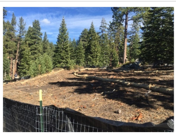
Foundation after filled in and graded to match original contour of the land. A seed mix of native vegetation was applied at the conclusion of grading.
